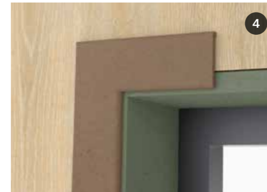
Window finish with MDF and window frame
