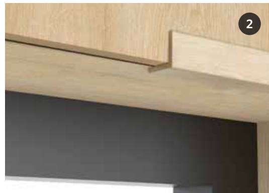
Window finish with flexible corner profile
