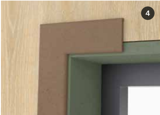
Window finish with MDF and window frame
